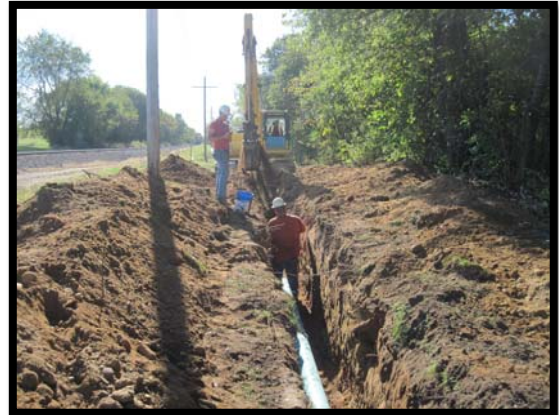
Zoarville Waterline Project
