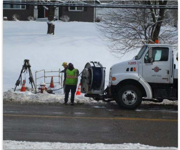
Mineral City Sewer Rehabilitation Project
